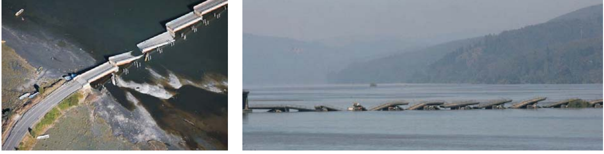
Figure 2: View of the destroyed “Puente Viejo” over the Biobio river, that links Concepcion and San Pedro de la Paz, 500 km south of Santiago, Chile, after the 8.8 magnitude earthquake on February 27, 2010. © Nicolás Piwonka, National Geographic.
